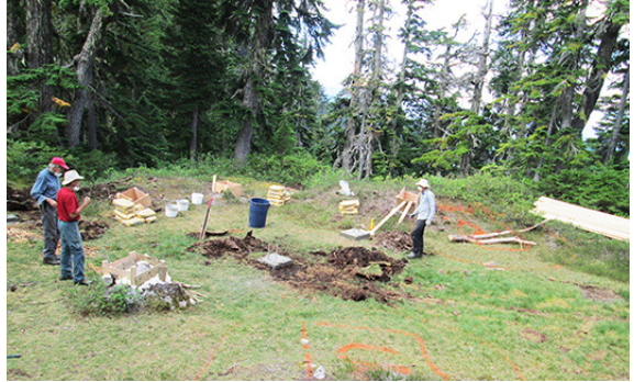
Finally, the foundations - in August, 2016. Photo: B. Wood.
